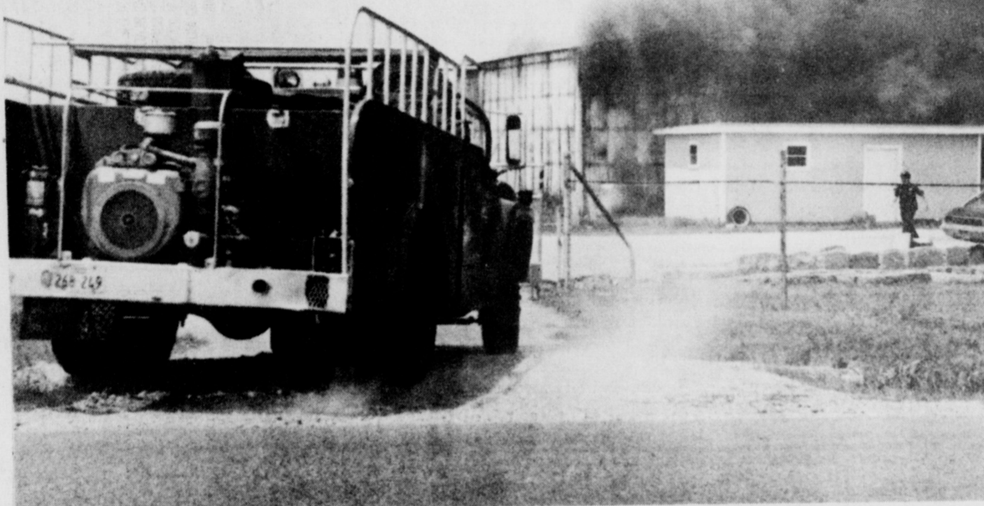
SAVED TWO STRUCTURES - Area volunteer firemen were unable to save a large metal building and its contents Tuesday afternoon, but were able to keep fire away from a wooden office building and a mobile home next to it. The structures belong to Wichita Monument Co., and are located at Bacon Switch Road and FM 369.
