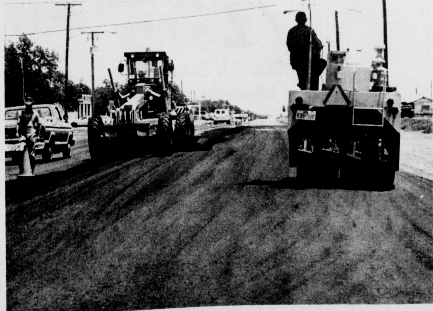
SMOOTH DRIVING - Highway Department personnel and equipment began last week and completed Tuesday resurfacing of East Highway, from Bell Road to Yosemite.
