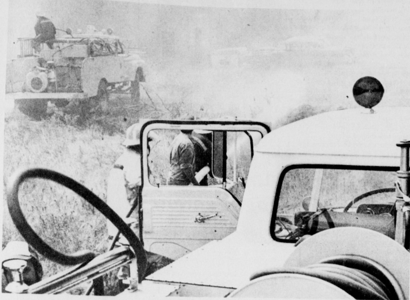
BURNING GRASS AND TREES threatened the homes on the south side of 800 block of Van Horn Friday afternoon. Firemen, however, were able to bring the blaze under
