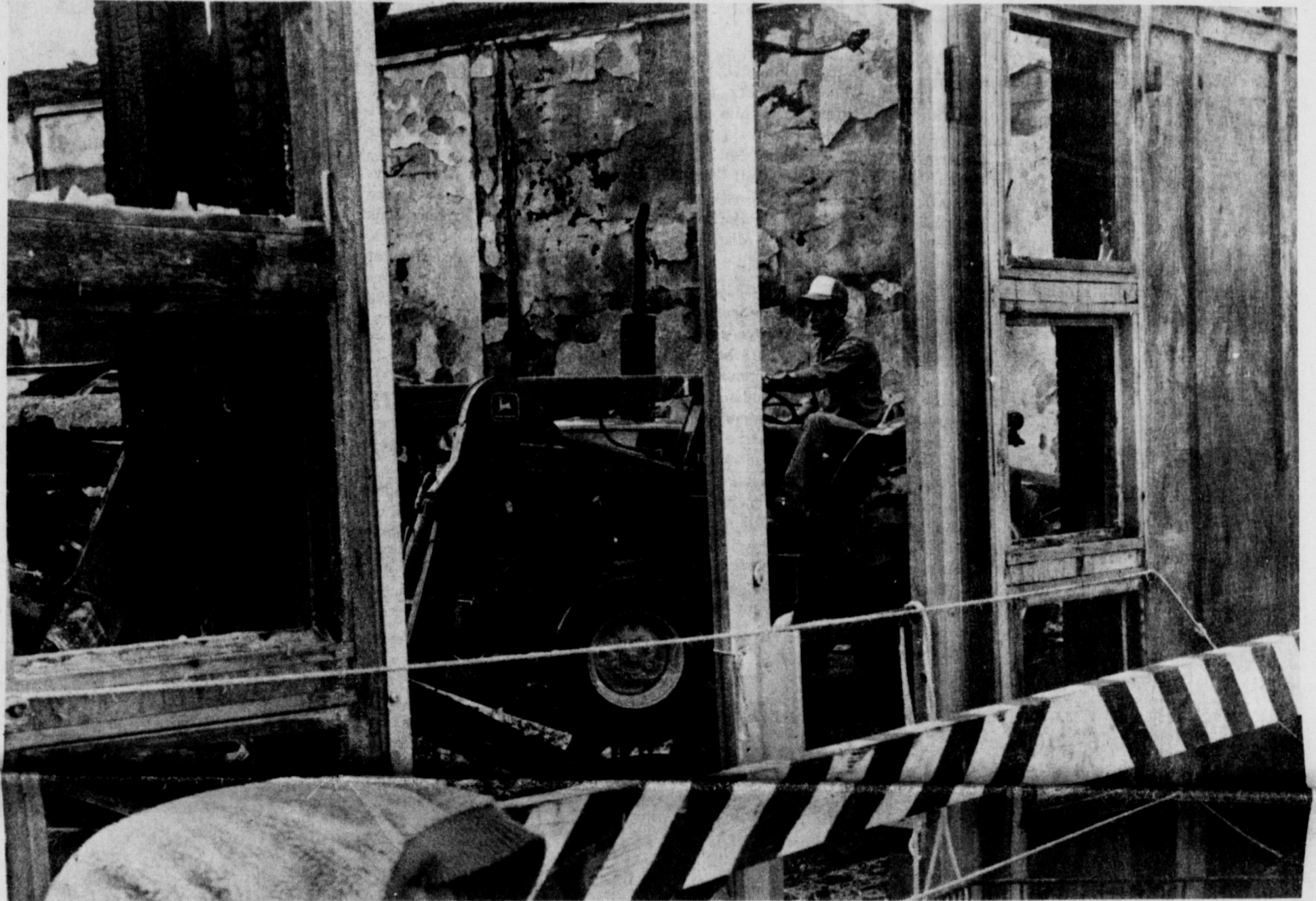
CLEANING-UP OPERATION BEGINS- Workers began this week cleaning up the burnt ruins of Discount Food and the Bee Hive. A steady stream of trucks were making the run between the site of the Dec. 8 fire and the city's sanitation
