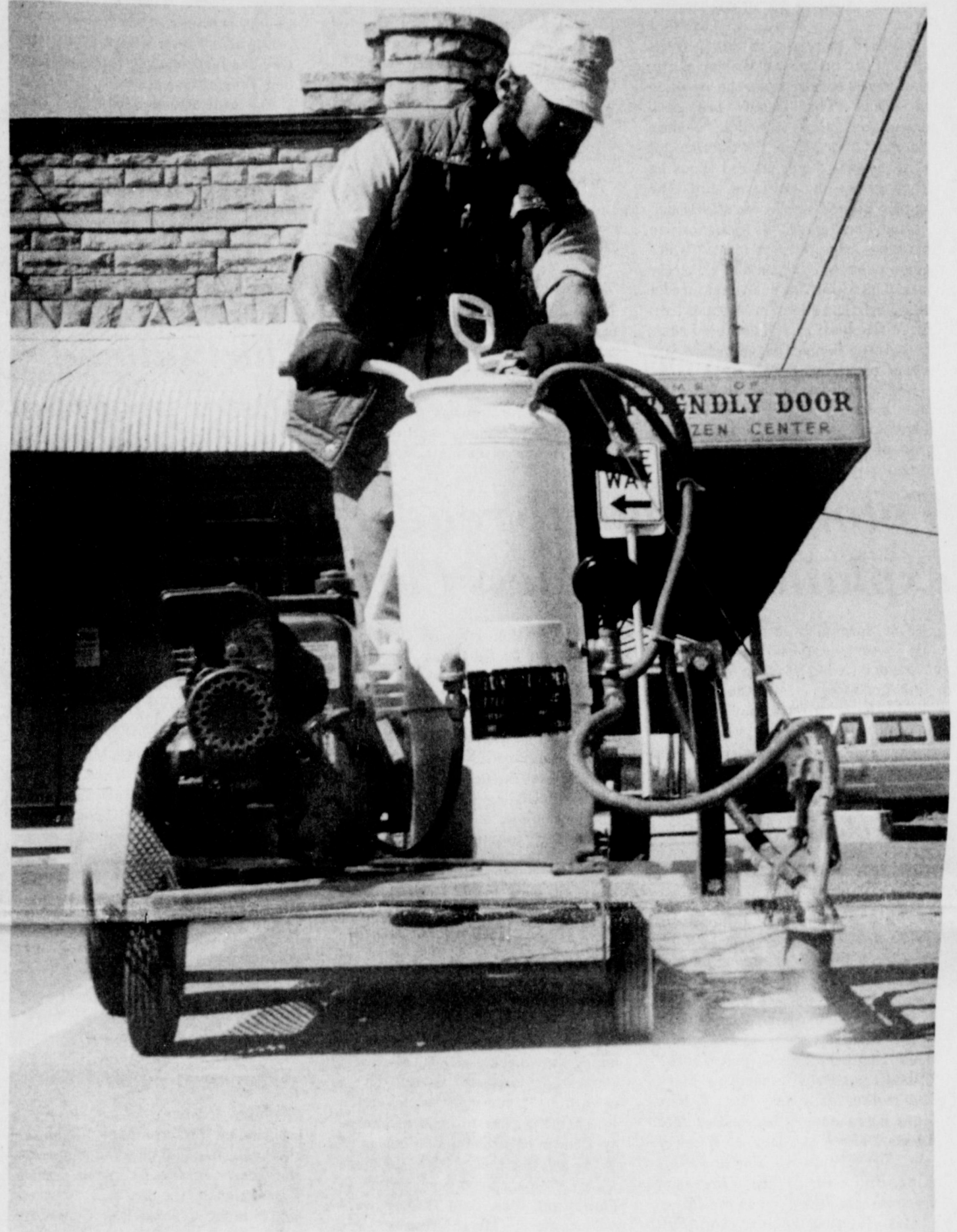
SPRING SPRUCING - City workman Mike Price paints walkway at the corner of Wall and Cash, as part of a project to designate traffic zones in the downtown area. Center
