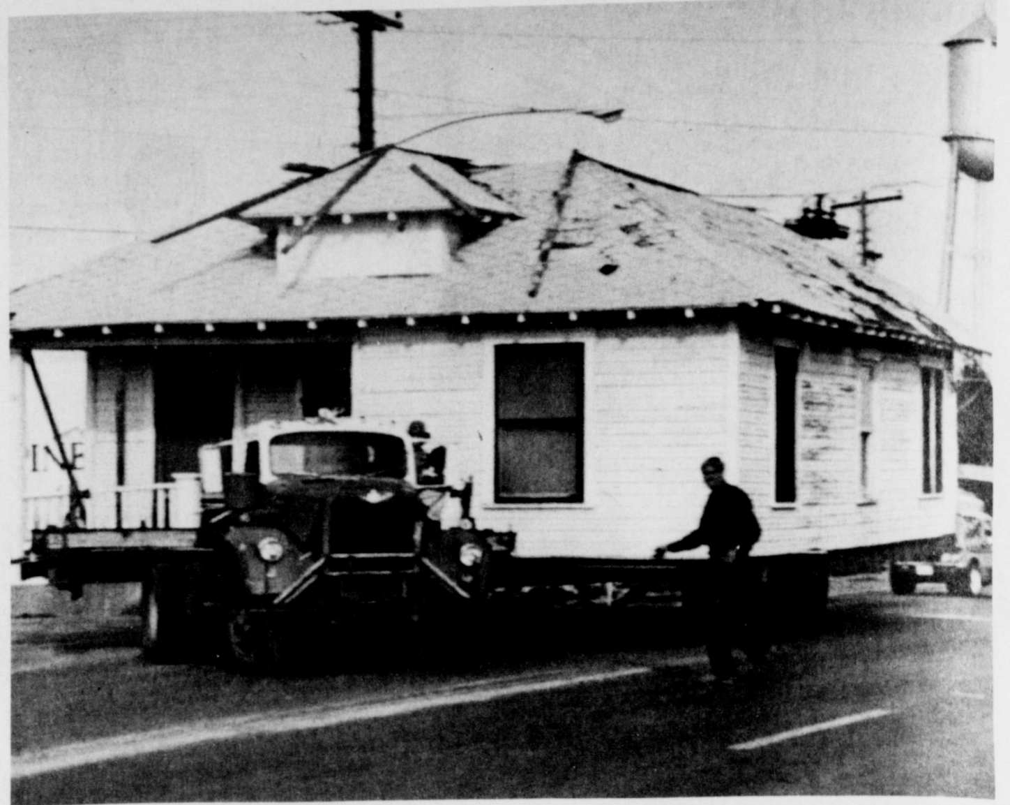
A TAD TOO TALL - Workers moving a home west on the Iowa Park Highway encountered a bit of resistance last week when the roof caught a signal light at the intersection
