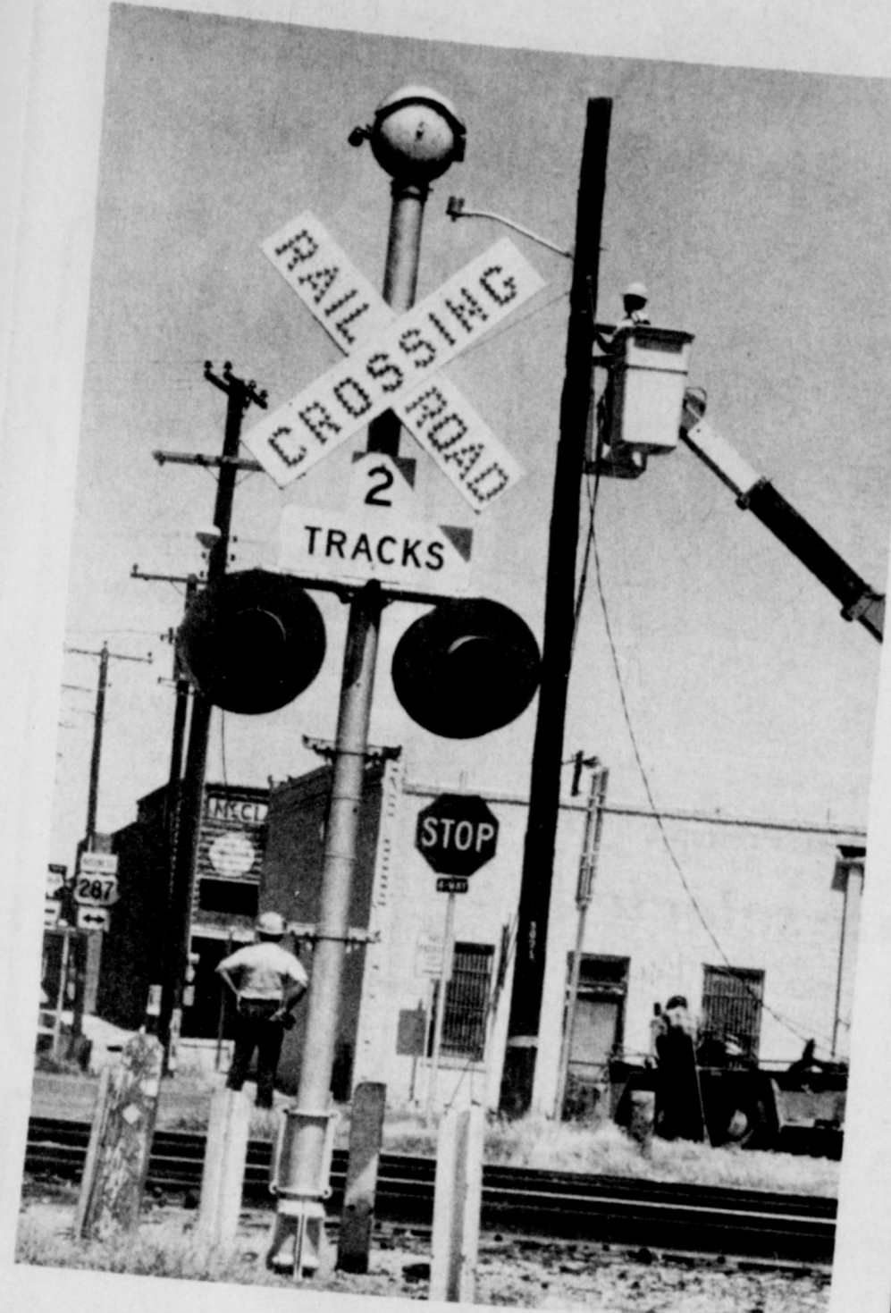
LIGHTED CROSSING - Workmen have been installing street lights at railroad crossings in the city to assist night drivers in seeing rail cars. The suggestion came from a state hearing held here last spring.
