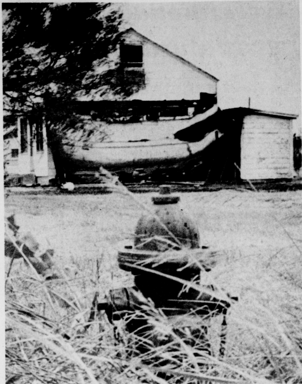
HEAVY DAMAGE was inflicted to the Ted Williams home, 202 E. Crystal, Saturday afternoon. Origin of the blaze has not yet been identified. Firemen could not use the fireplug in the foreground, apparently because of a faulty valve, and had to use another plug nearby.
