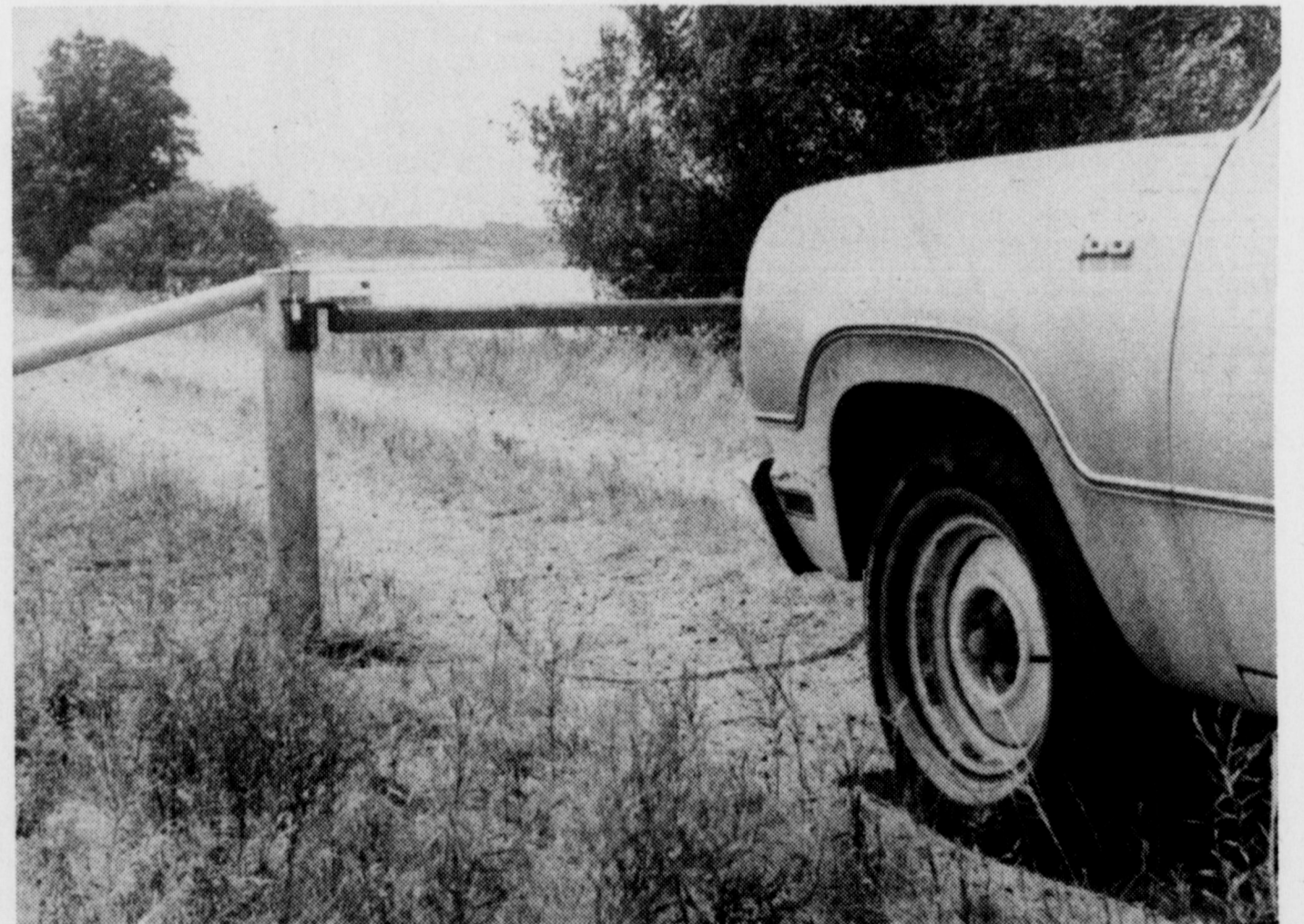
REPAIRED BARRIERS, WITH LOCKS, TO STOP DRIVING ON LAKE DAMS ...city council sets $100 fine for violations
