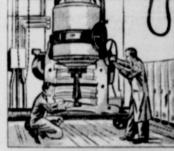
A regular check-up on pieces of 4. X-ray exposure needed for 5-X-ray film worn on workers' wrists inch-thick steel is now 2 minutes helps guard against prolonged instead of previous 3½ hours! exposure to the rays given off by the X-ray tube. Whole days are saved in examina tion of even thicker castings.
