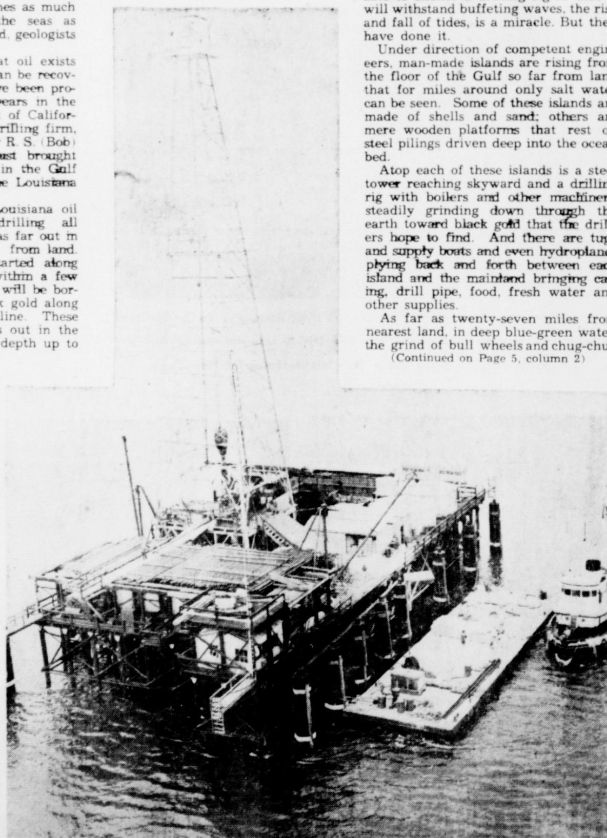
DRILLING FOR OIL IN GULF OF MEXICO . . . This oil well was drilled 20 miles from land, in the Gulf of Mexico, in water 20 feet deep, by the Magnolia Petroleum Co. Drilled to a depth of 12,874 feet, it was a dry hole.
