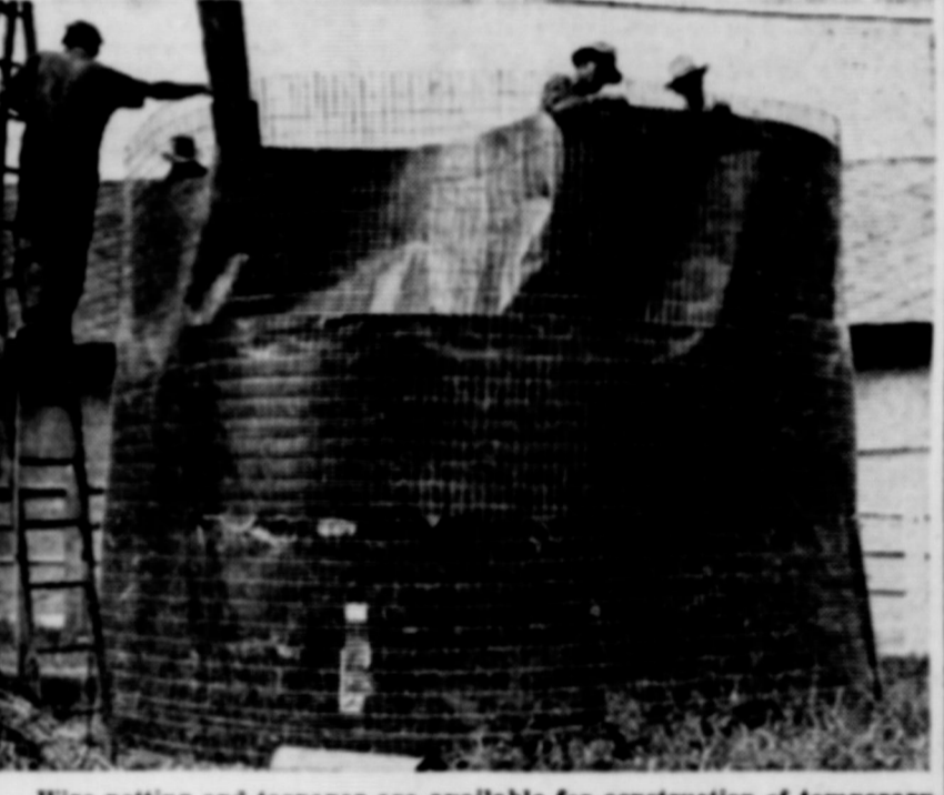
Wire netting and tarpaper are available for construction of temporary storage bins such as this one. It is necessary, however, for farmers to apply to dealers well ahead of time, as supplies are limited.
