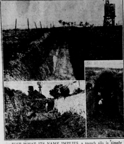
JUST WHAT ITS NAME IMPLIES, a trench silo is simply a trench dug into the ground into which chopped feed crops may be stored for feeding as succulent ensilage to dairy cows, best cattle and work stock during periods of dry pastures or bad weather. Cheap, easily dug, easily filled, ensilage easily removed, the big disadvantage of a trench silo is excessive spoilage which may be avoided by properly filling, and by providing drainage. More than 200 were dug in Texas in 1931 and county agent reports indicate a big increase for 1932, especially in West Texas.
