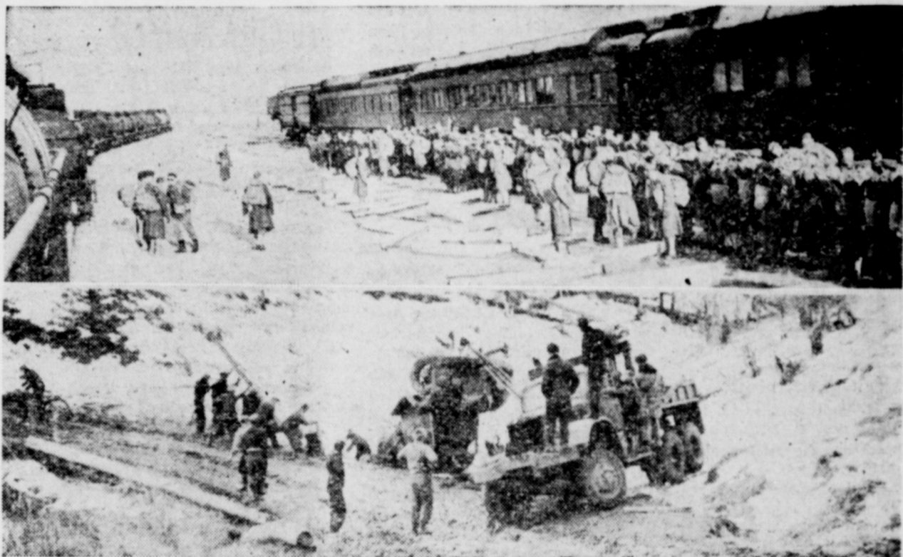
Upper picture shows journey's end, as U. S. engineer corps troops arrive at the end of the steel ribbon, at Dawson Creek, B. C., to start building a highway to Alaska from the end of the present road at Fort St. John. Below: First activity of road building at start of construction of the Alaska highway. Note men in foreground with truck pulling another road-building truck out of a ditch. All equipment for the project was shipped from the States.
