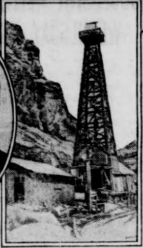
Just Room for the Derrick
