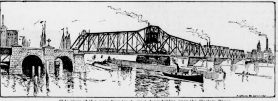
Side view of the new four-track steel draw-bridge over the Harlem River.
