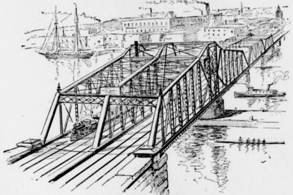
End View of the New York Central's new four-track steel draw-bridge over the Harlem River at 151st Street, Greater New York. The largest structure of its kind in the world.
