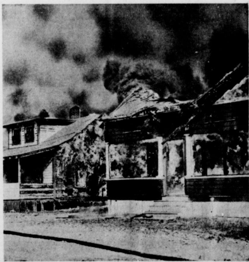
Damage estimated at about $2,000,000 was caused in the Ocean Bluffs, Mass., area as the result of a fire that destroyed a church and leveled more than 450 cottages. Only a timely shift in wind saved hundreds of other houses. The above photo shows a row of cottages burning fiercely when the fire was at its height.
