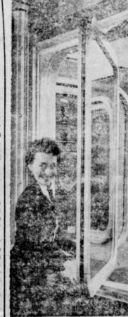
WASHING WINDOWS of the ultra-modern Alcoa Building in Pittsburgh, Pa., has been simwindows at Alcoa means deflat-ing the butyl tube, swinging the win ow in ide the building for win ow ir ide the building for cleaning, then swing in it back into posi on. The tube, designed by the General in & Rubber Compiny, hilds the wir ow in pice. No longer need the wincow-washer dangle precariously 1 om the 42-foor win ow casing. His is now an inside job.
