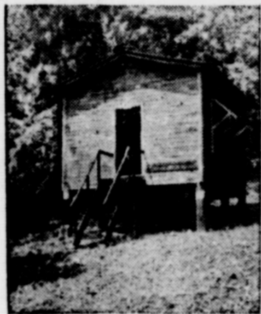
Panama test house. This photo shows that treated wood had not been attacked by termites.
