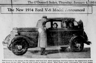
Refinements in the design of the radiator and hood and more luxurious interiors feature the appearance of the new Ford V-S for 1934. The de luxe Tudor is shown above. Dual down draft carburetion and dual intake manifold give the engine greater power, the car increased pickup and speed. A clear-vision body ventilation system also is introduced in the new Fords.
