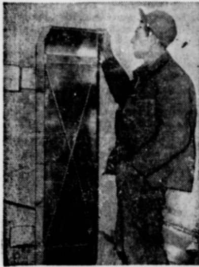
Arthur Miller of Union, Ill., admires the new heater recently installed in his milk house.
