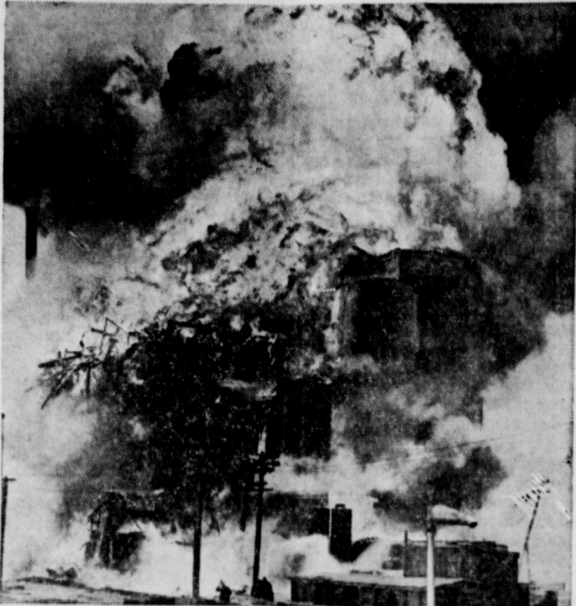
This spectacular picture was taken just as a billow of white hot flame blew off the top of a United States Grain elevator, in Chicago, during a $300,000 fire, of mysterious origin. More than 350,000 bushels of corn were destroyed. Furnace-like heat melted steel girders like butter and drove back firemen.
