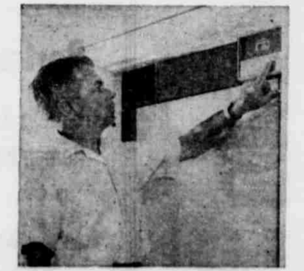
Mr. Sims points out the simple control on the electric air purifier which automatically rejects pollen, dust and other irritants, giving the Sims family clean, fresh air throughout the home.
