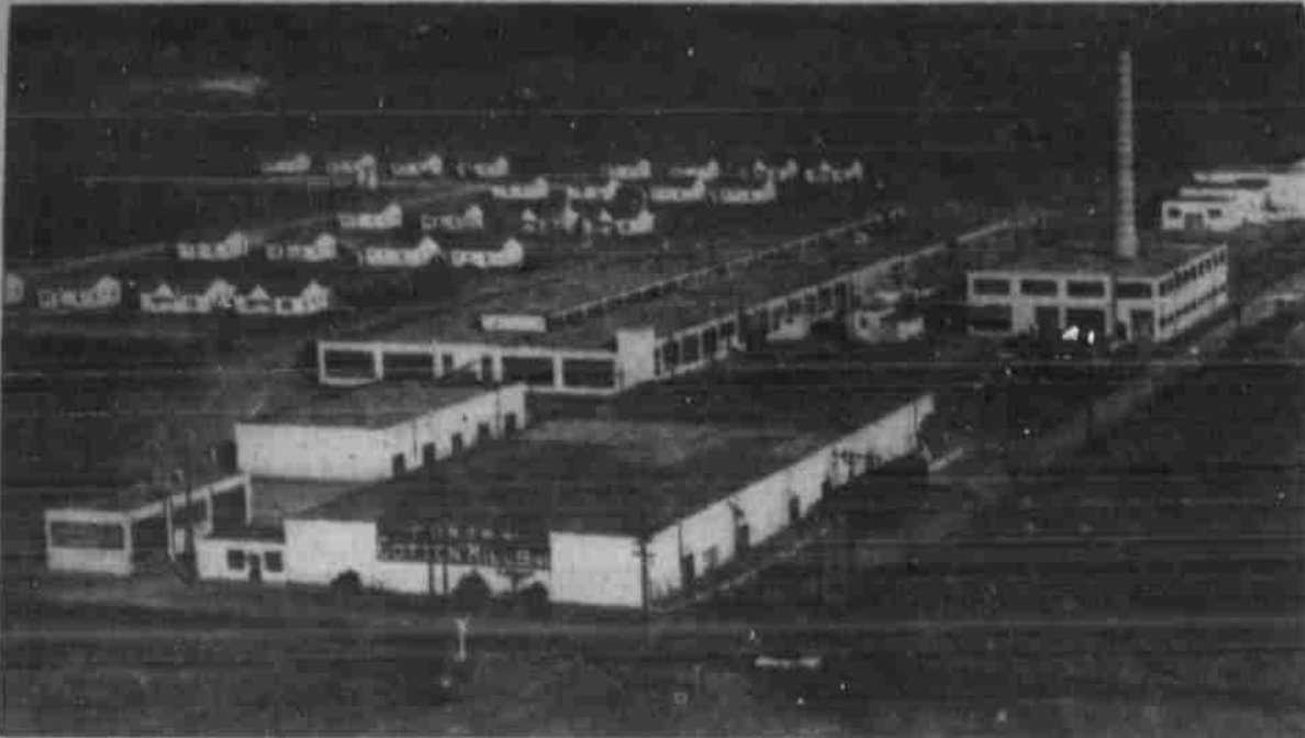
AERIAL VIEW OF MILL—This is an aerial shot of the original Postex Mills, as built by C. W. Post to market the cotton grown in the area. The plant has been greatly expanded through the years, the most recent program being a 1956 project costing more than $1,000,000.
