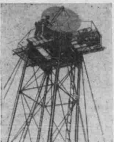
STORM RADAR — Wash., D.C. — Two Signal Corps soldiers set up a portable storm radar, the Army's new weather eye for spotting significant storms at distances of 200 miles. The 25-foot tower can be set up in a day to allow Army scientists to predict within minutes when a storm will strike any spot within range.
