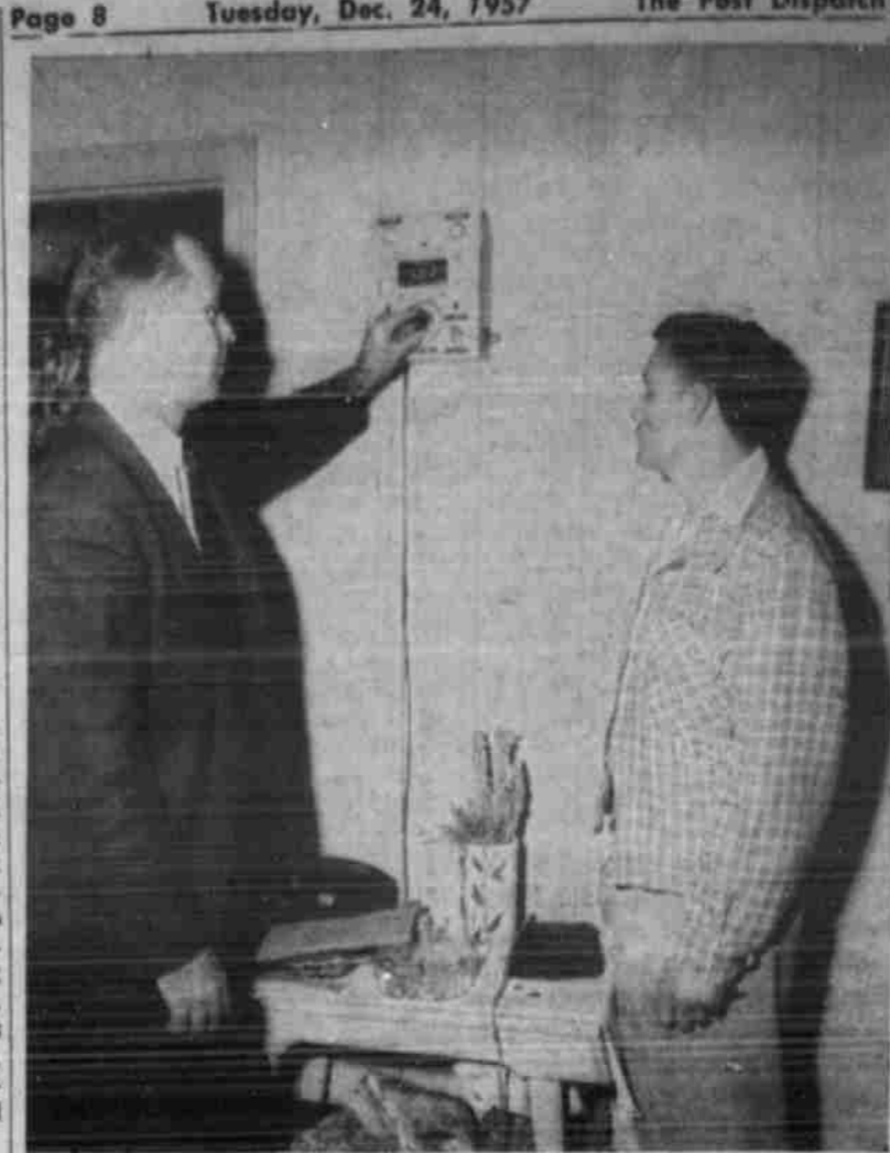
PRESSURE INDICATOR INSTALLED — Meteorologist Jim White (left) is explaining to Rufus Gerner of Mason Funeral Home the operation of a pressure jump indicator installed by the U. S. Weather Bureau at the funeral home. The indicator will make it possible for the weather station at Amarillo to anticipate areas of possible severe weather in the Post vicinity.—(Staff Photo).
