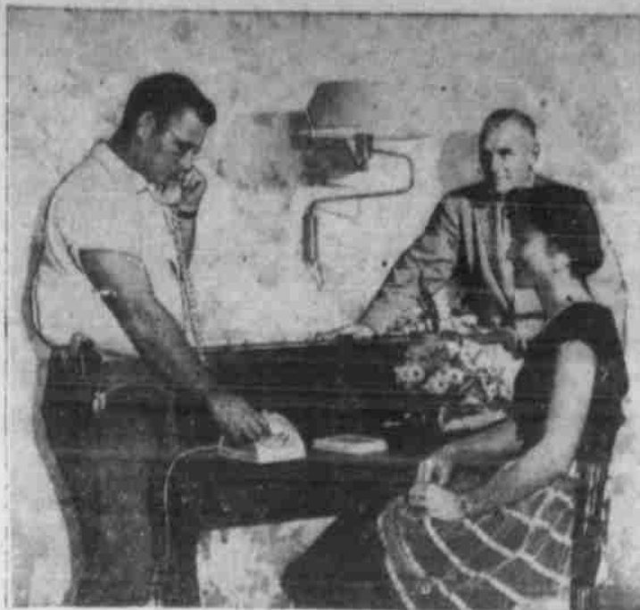
QUARTER-MILLIONTH TELEPHONE — G. Howard Briggs, operating vice president for General Telephone Company of the Southwest, looks on as General's 250,000th telephone is installed in the home of Mrs. R. E. Kane of Denton, Texas. James M. Glover, installer repairman at Denton, is shown testing the instrument before Mrs. Kane makes the first call on the new yellow extension telephone. General is the largest independent (non-Bell) telephone company in the Southwest and operates 264 exchanges in Texas, New Mexico, Oklahoma, Arkansas and Louisiana.
