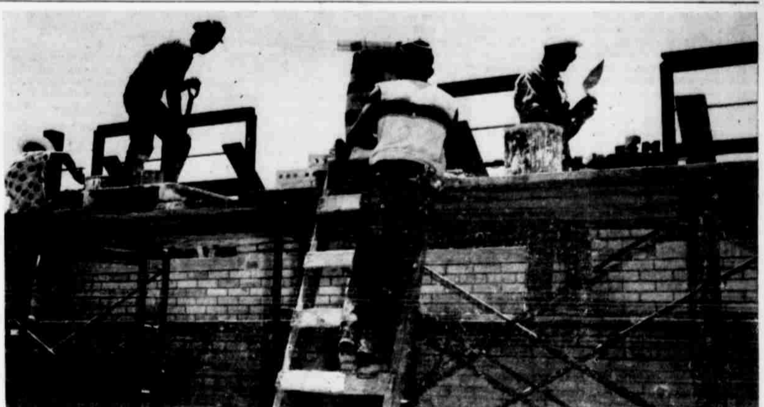
SCHOOL WALLS GOING UP—Temporarily delayed last spring because of non-arrival of materials, brick work is now proceeding at a rapid pace on the new junior high school building. Workmen are shown here at work on the gymnasium wall.
