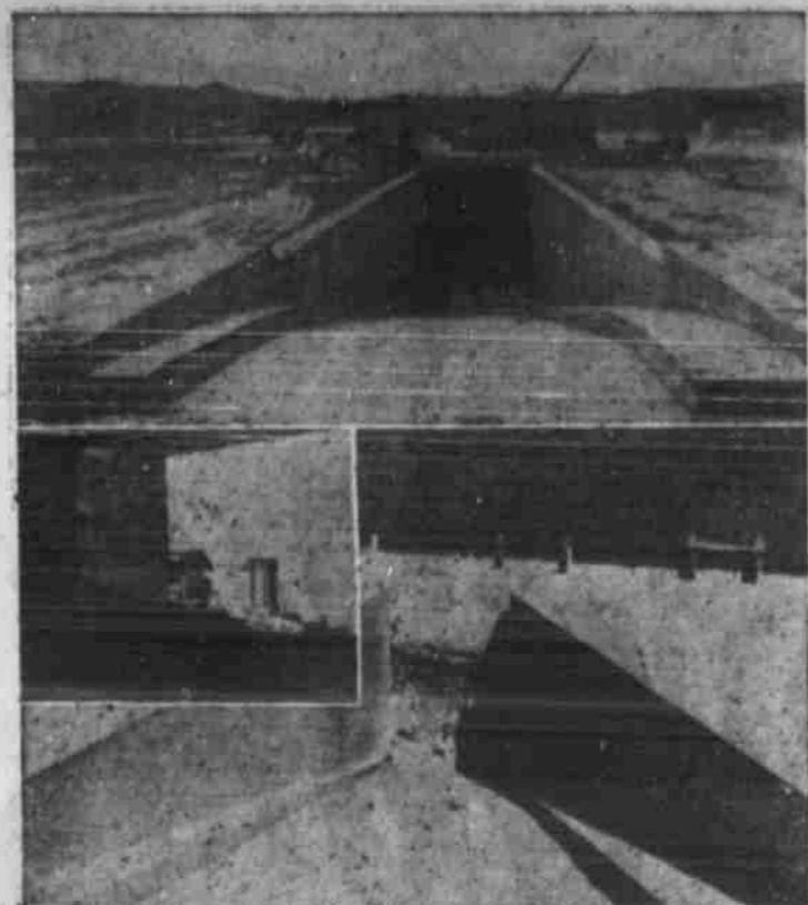
AUTO ENTRANCE ramp burrows inconspicuously into the desert as it leads down to a dual-purpose underground shelter and garage at the Operation Plumbob atomic tests in Nevada. Lower photo shows how the A-bomb blast crumbled part of the concrete retaining wall but failed to block the entrance. To the right of the crumbled wall is the entrance, closed by a 100-ton, four-foot-thick reinforced concrete blast door (inset), which was undamaged. (GPO Lookout Mountain Lab Photo)
