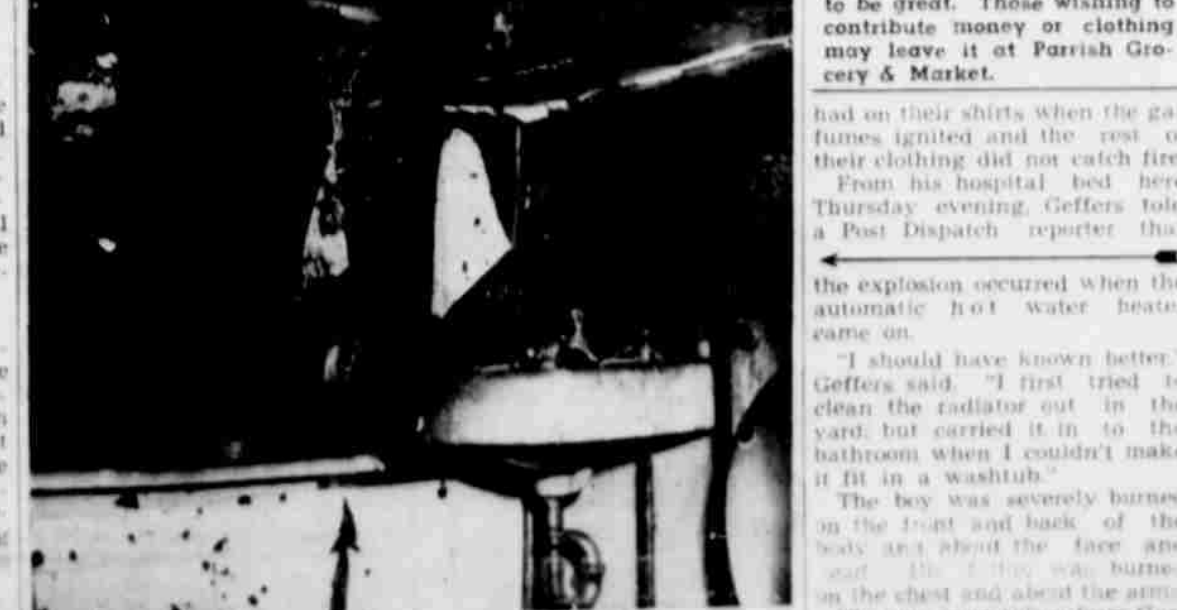
EXPLOSION SCENE —This is a view of the bathroom at the Paul Geffers, Sr., home following a gasoline explosion which burned four members of the family, one critically. (Staff Photo)
