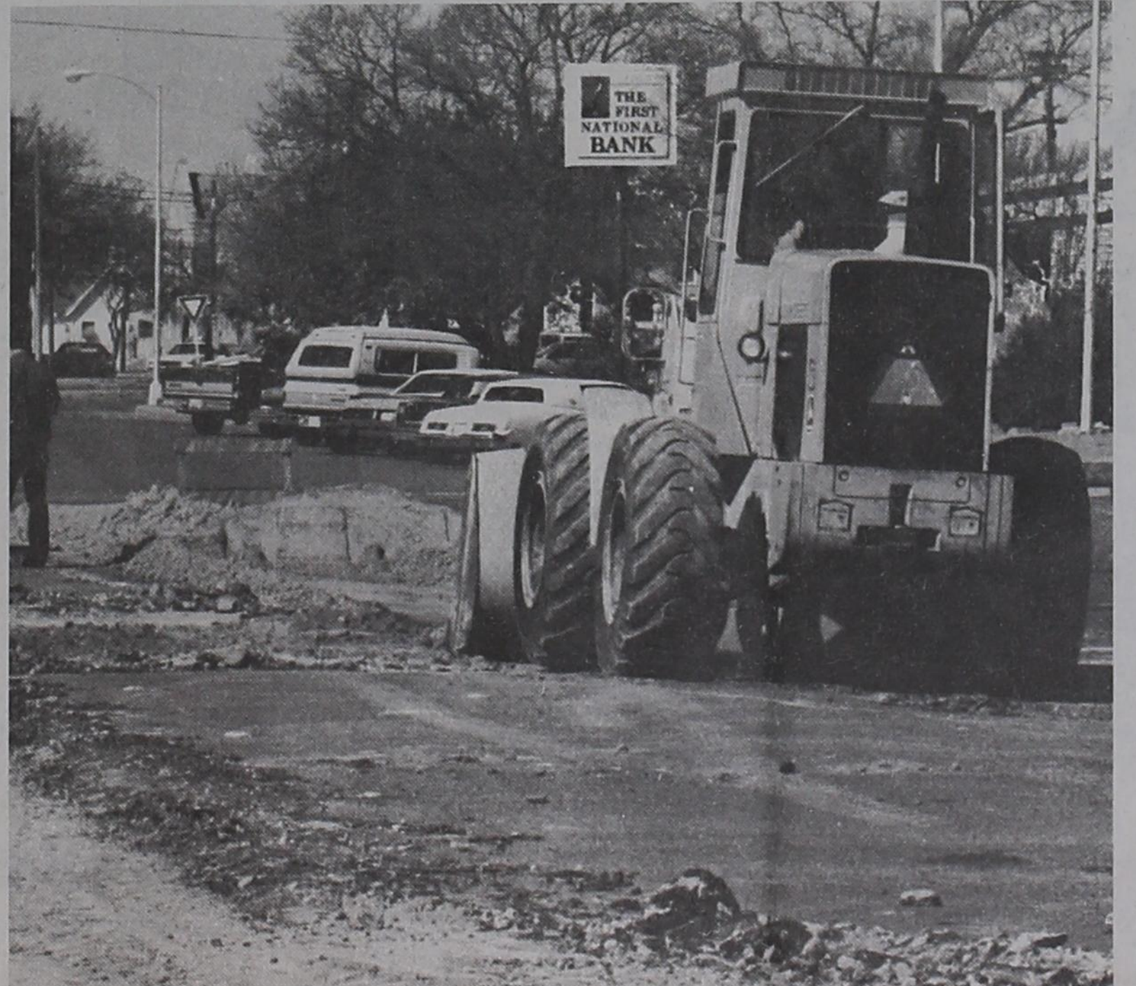
WEST MAIN STREET reconstruction began Monday as city and county crews broke the old asphalt in the center of the street. The landscaping project will match the work completed last year on East Main Street. The new project is funded by private donations.
