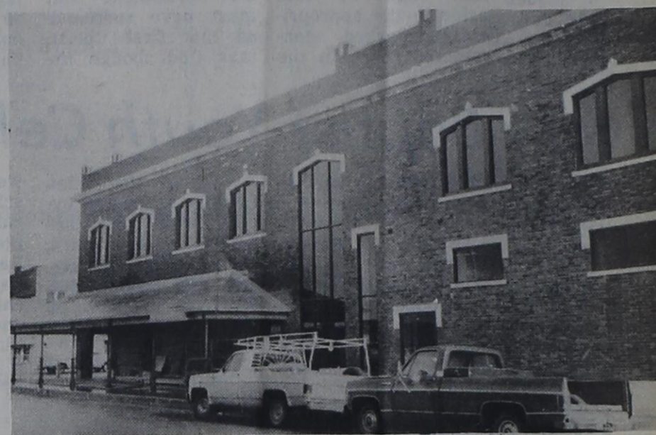
Giles McCrary's restoration work at the Double U Building.
