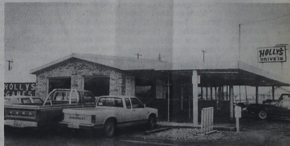
Lewis Holly's recently remodelled facility.
