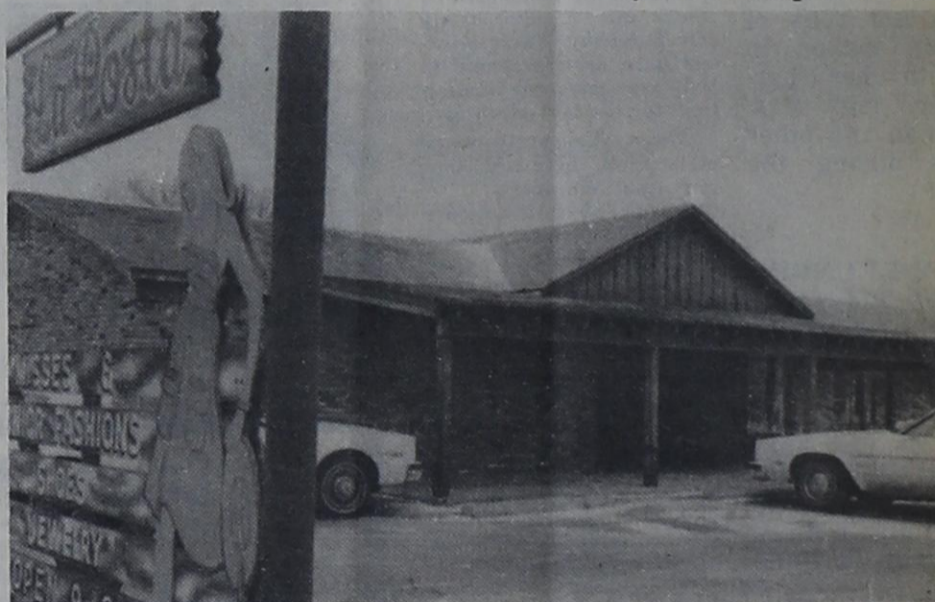
Ada Lou Bird's expansion and remodelling at La Posta.
