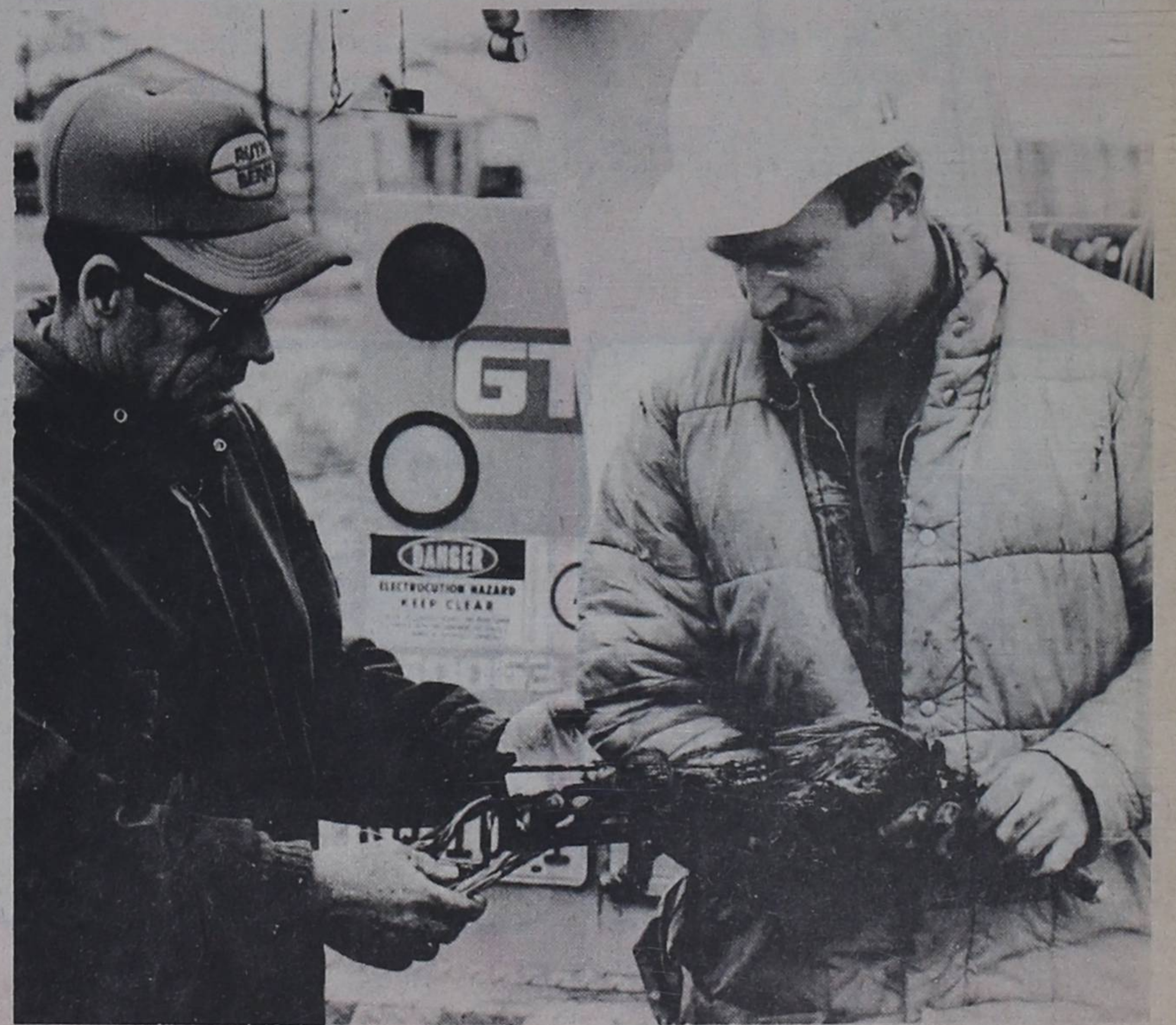
A. J. Baumann, combination man-in-charge of GTE's Post office, inspects the remains of a 200 pair burned telephone cable on South Ave. O with Danny Stancell, GTE cable
