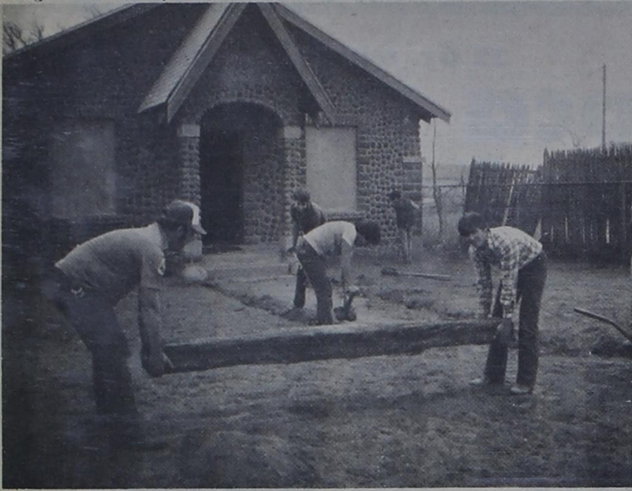
LIFTING AND SHOVELING — Shown above are Scoutmaster Jerry Stegall, far left, and members of Boy Scout Troop 316, as they were landscaping the yard at their new meeting place, the old American Legion Hall. Shown above are Wayne Smith on the other end of the cross-tie and center front, Bobby Garcia, Jimmy Ticer and Wade Smith. Not pictured were Bobby Smith, Kelly Binford and Dicky Odom. (Staff Photo)
