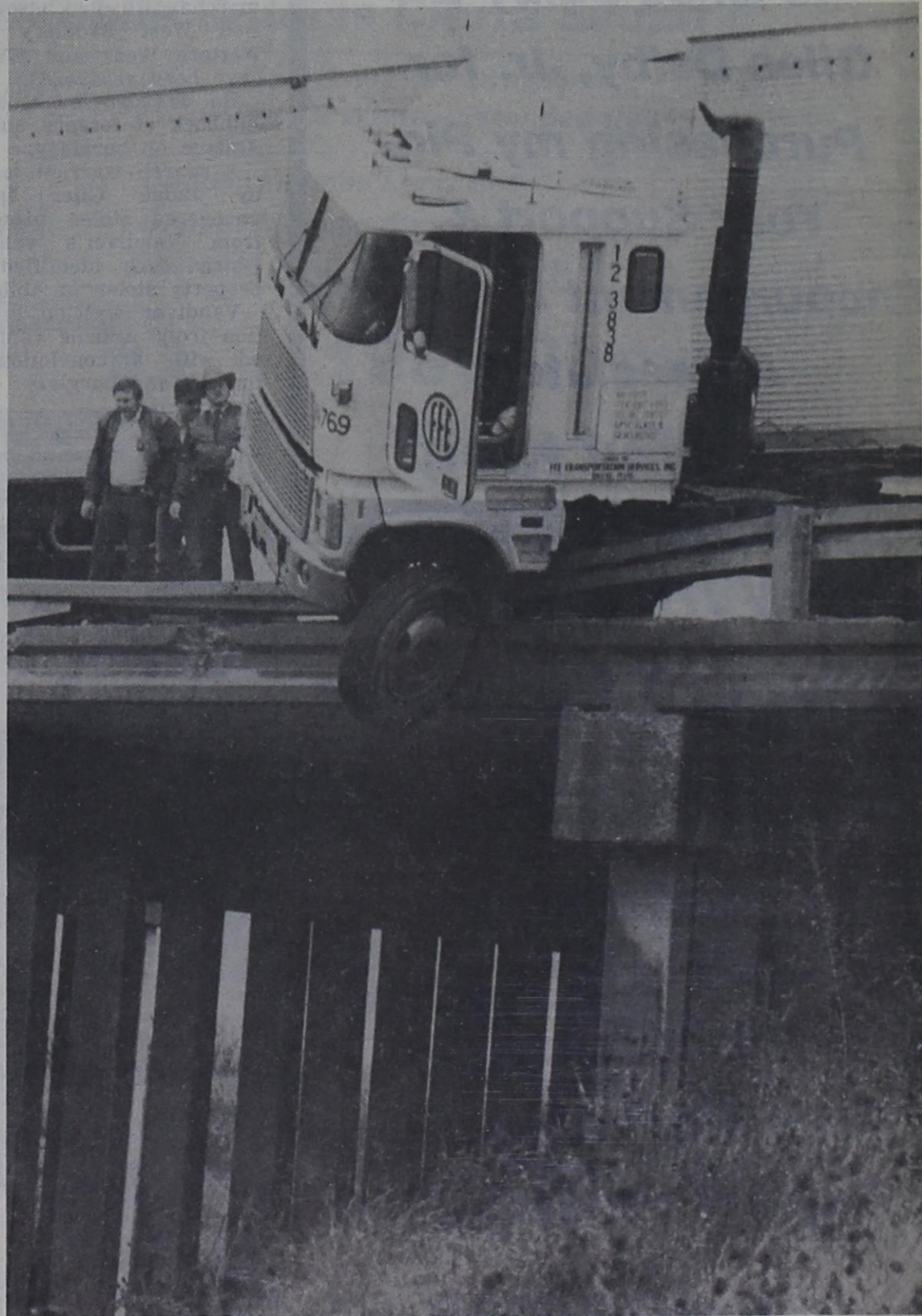
A CLOSE CALL - Truck driver L.C. McDaniel of Fort Worth came a few inches from falling with his cab over the U.S. Hwy 84 railroad overpass south of Post last week. The rain-slicked highway resulted in the vehicle jack-knifing, hitting the rail and breaking the guard rail. McDaniel was able to climb out uninjured.
