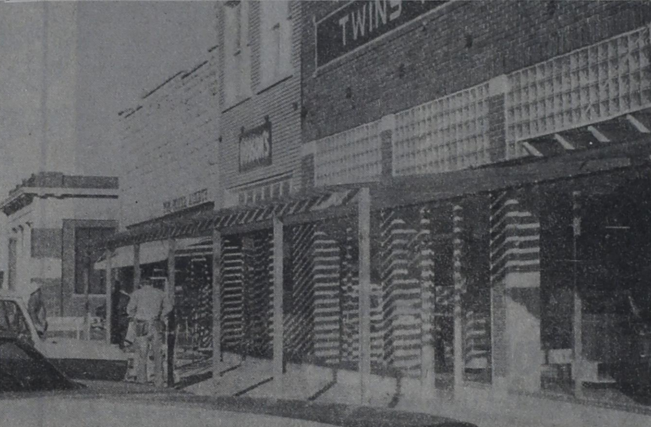
DOWNTOWN RENOVATING — Businesses and building owners on the north side of East Main in Post are sprucing up building fronts as part of a revitalization campaign.
