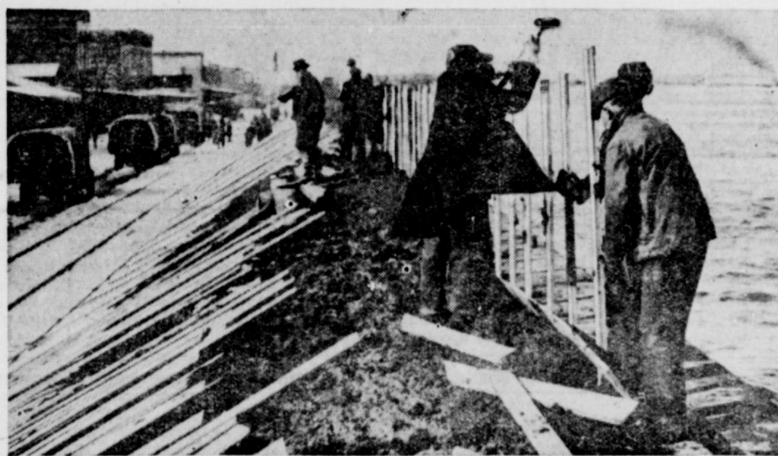
Workmen are pictured building up the Mississippi river levee at Cairo, Ill., in an effort to stem the rising waters. The most disastrous flood in the history of the father of waters cost hundreds of lives, rendered more than a million people homeless and caused hundreds of dollars worth of damage.
