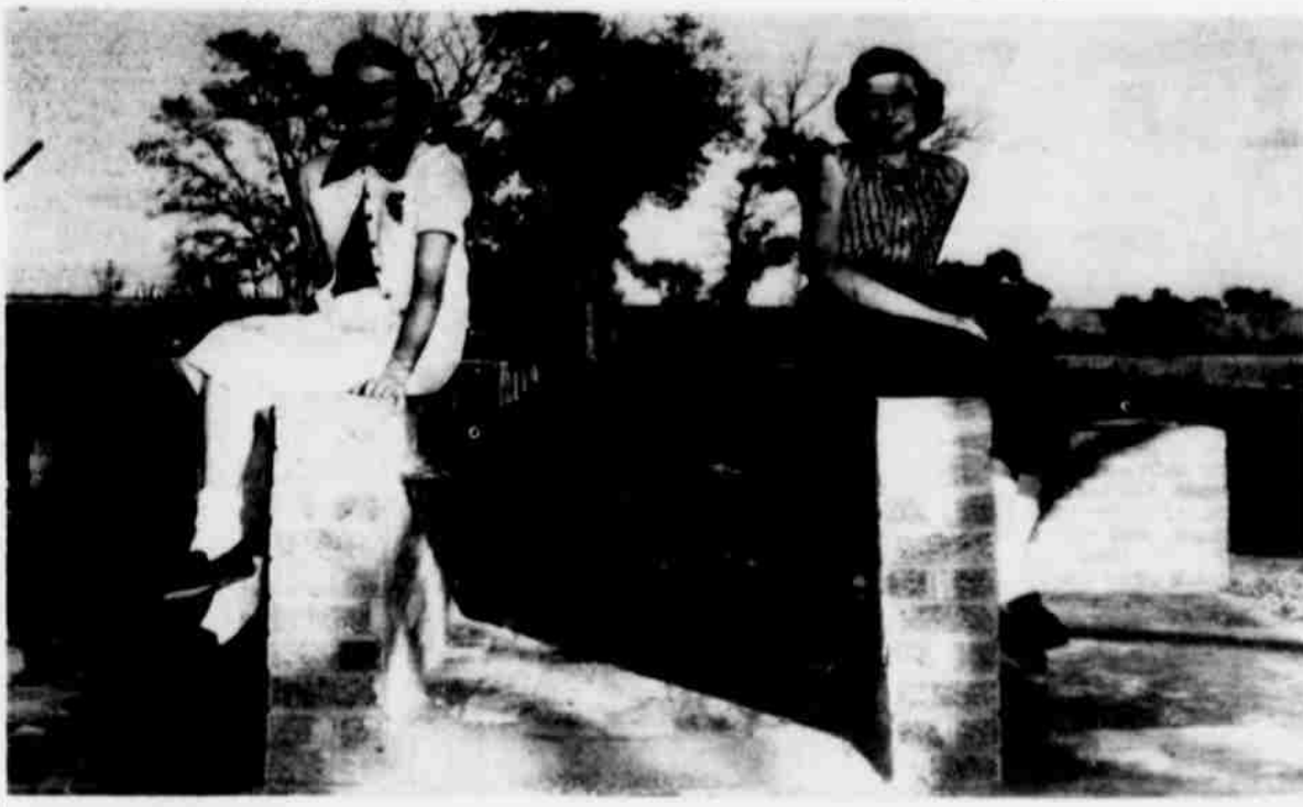
PARK PROJECT NO. 1—This barbecue pit, construction of which was made possible by an anonymous donor, was completed recently at the City Park site by George "Scotty" Samson. Two of the many admirers of the attractively-constructed pit are Miss Carolyn Hudman (left), daughter of Mr. and Mrs. Marvin Hudman, and Miss Mary Lou Hedgepath, daughter of Mr. and Mrs. G. E. Hedgepath.—(Staff Photo).
