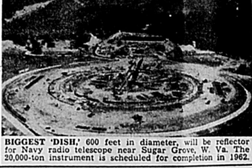
BIGGEST 'DISH' , 600 feet in diameter, will be reflector for Navy radio telescope near Sugar Grove, W. Va. The 20,000-ton instrument is scheduled for completion in 1962.
