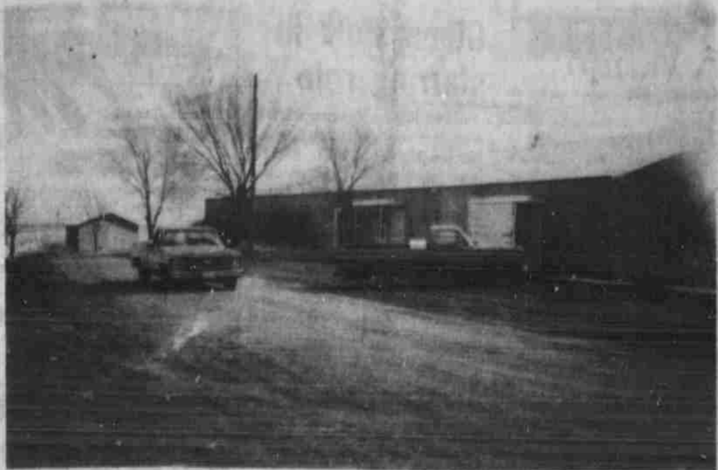
THIS WAY OUT — A new road has been built around the 4-H building with the exit made on the north side of the building which should help ease the traffic flow to and from the area. A few parking facilities have been made in front of the fair building area to enable the ladies working there to unload more easily. — (Staff Photo)
