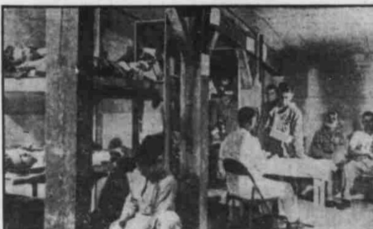
A three-ward underground hospital, complete with X-ray equipment and facilities for operating was dug out of the sandstone and solid rock at Camp Joseph T. Robinson, Ark.
