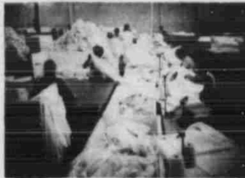
SEWING AND PACKING — The finished cloth is cut, hemmed and labeled for fitted sheets, flat sheets, and pillow cases. They are then inspected and folded in preparation for packing.
