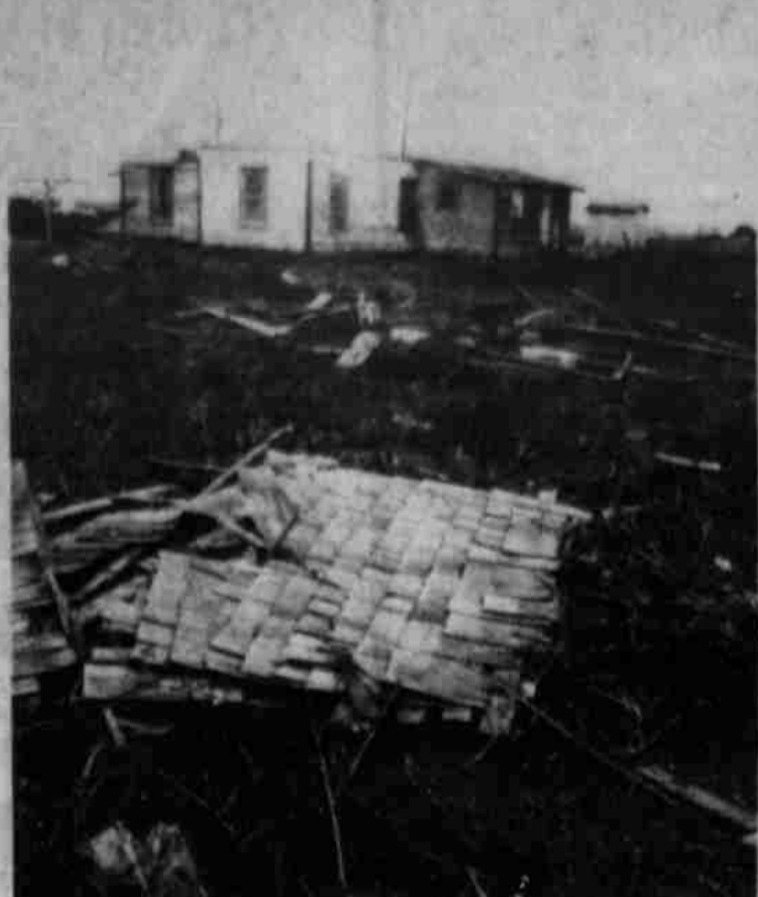
TORNADO DAMAGE — Shown left is the unroofed old Scott Storie farm home west of Post Sunday after it was hit by a small twister Saturday night. Most of the roof lies in the foreground. In the
