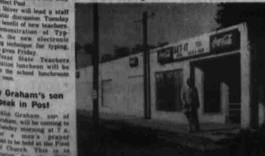
EYESORE TO GO — Allsup's Area Supervisor Stoney Stalcup stands at the entrance of the empty business building in the 400 block North Broadway which soon will be demolished to make way for a new Allsup Convenience Store on the site. The building was damaged by fire some years ago and never repaired.
