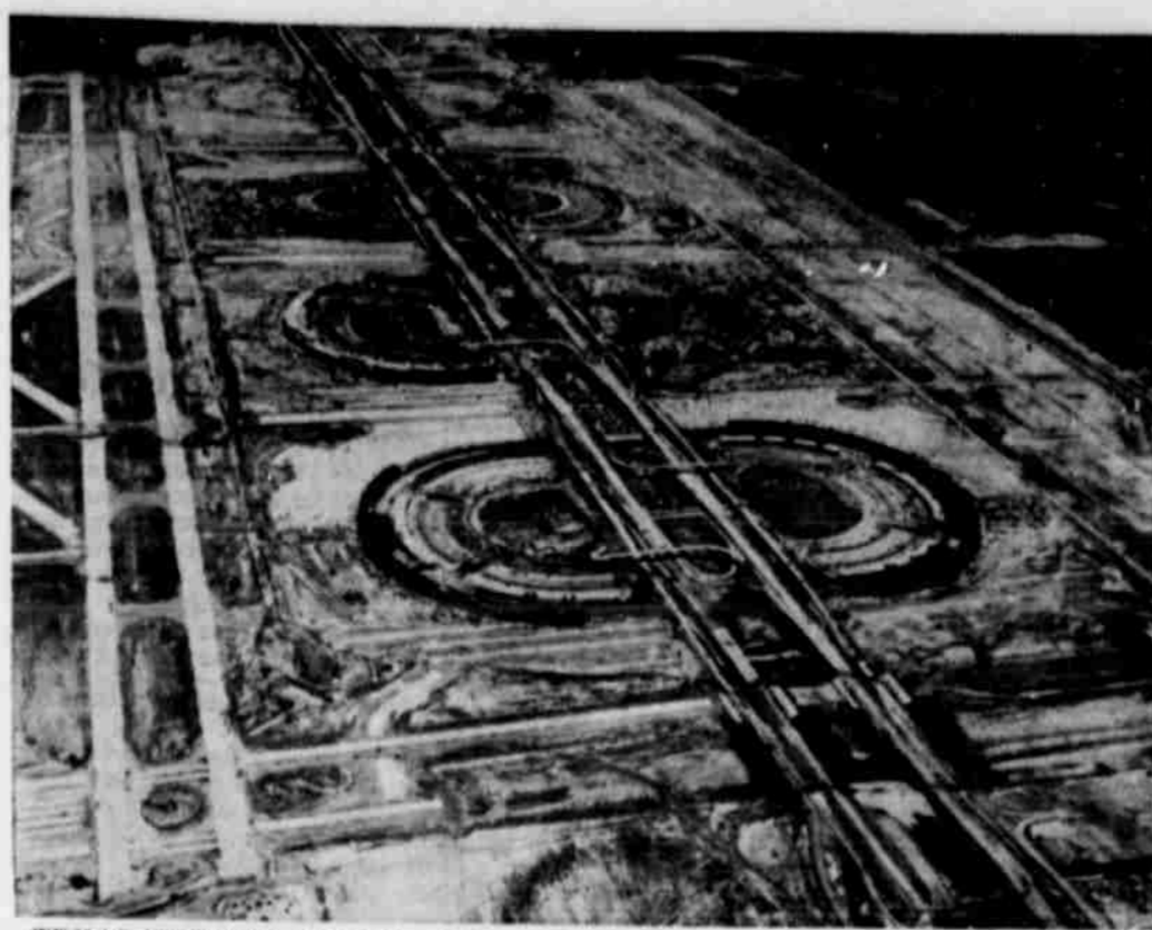
TEXAS-SIZE SUPERPORT — This aerial view of the new Dallas/Fort Worth Airport shows construction progress on the giant superport scheduled for opening in early fall, 1973. Conveniently located 17 miles from both Dallas and Fort Worth, the new airport is designed with the passenger in mind. Drive to gate boarding, close-in parking and simplified terminal procedures are only a few of the ultra modern features designed into the unique facility.
