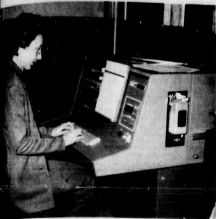
PHOTO-COMPOSITION —Bonnie Duren, Dispatch woman's editor, is at the keyboard of the CompuWriter, which sets the type for the columns, and also larger sizes, by photo-composition.
