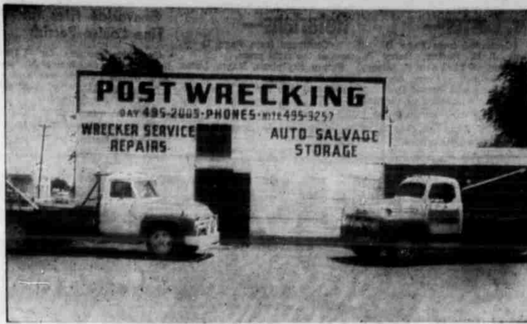
EXPANDED POST WRECKING CO. BUILDING Pictured above is the west front of the building of the Post Wrecking Co. at 201 South Avenue I, together with the firm's two wreckers which provide 24-hour, state-wide wrecker service. The building was remodeled and enlarged in 1963.—(Staff Photo)
