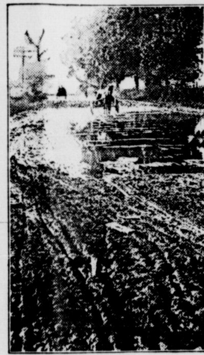
Stretch of Missouri Road Previous to Reclamation.
