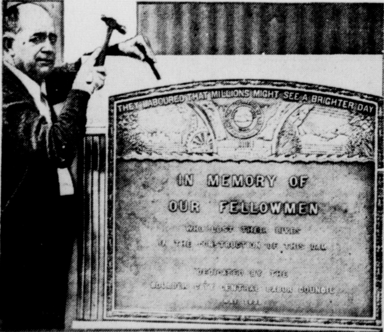
Wiley Rabun putting the finishing touches to the bronze plaque which has been set in the Nevada canyon wall near Boulder dam as a memorial for the men who have lost their lives in the construction of that great project.
