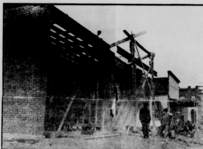
A Building under Course of Construction on South Main street
