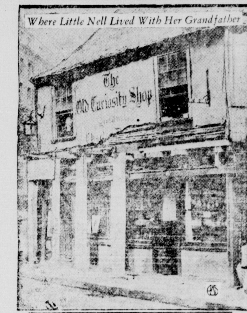
The Old Curiosity Shop, in London, made famous by Charles Dickens, is being repaired without changing its general appearance.
